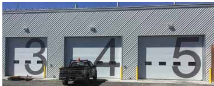
Energex Mark IV-200 - Salluit Airport, Nunavik
