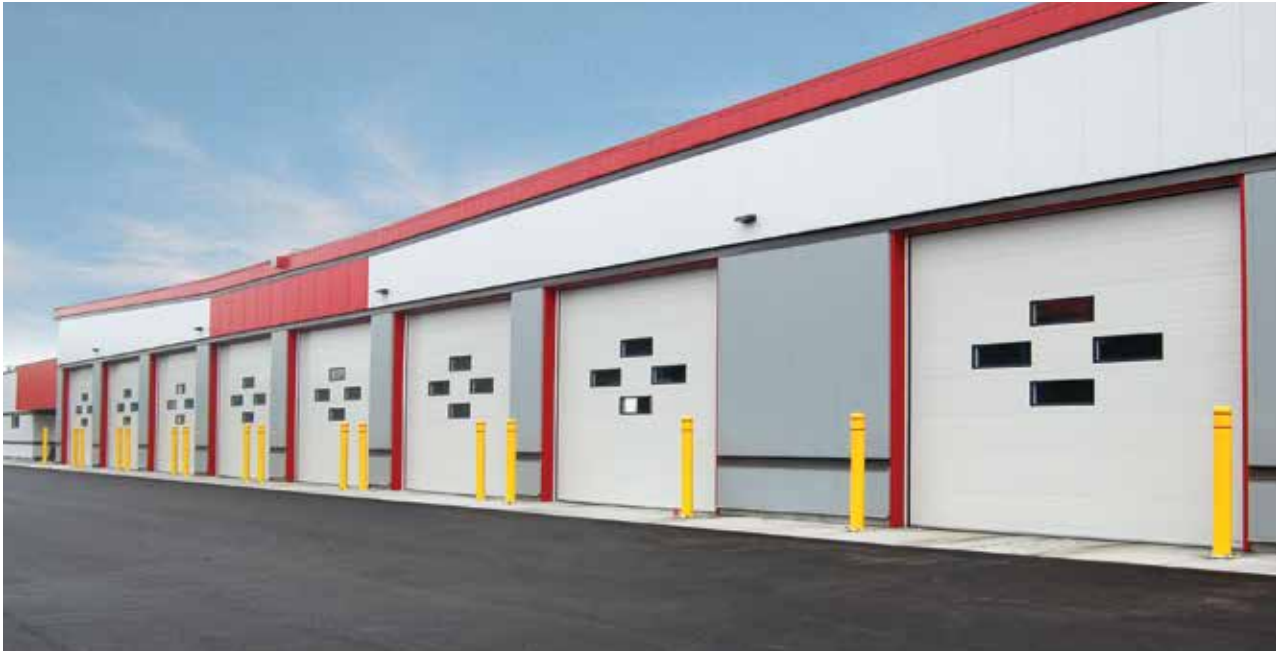
Energex Mark IV-200 - Municipal Work Yard, Ottawa, Ontario
